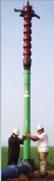
PPS During Installation
